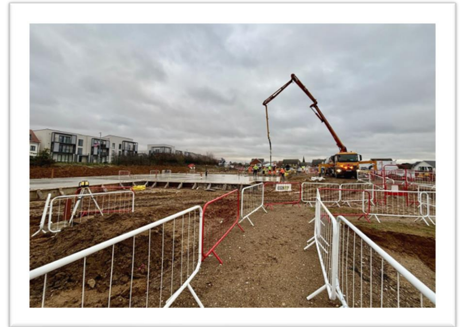
New 2FE NZ Primary School - Harlowbury
